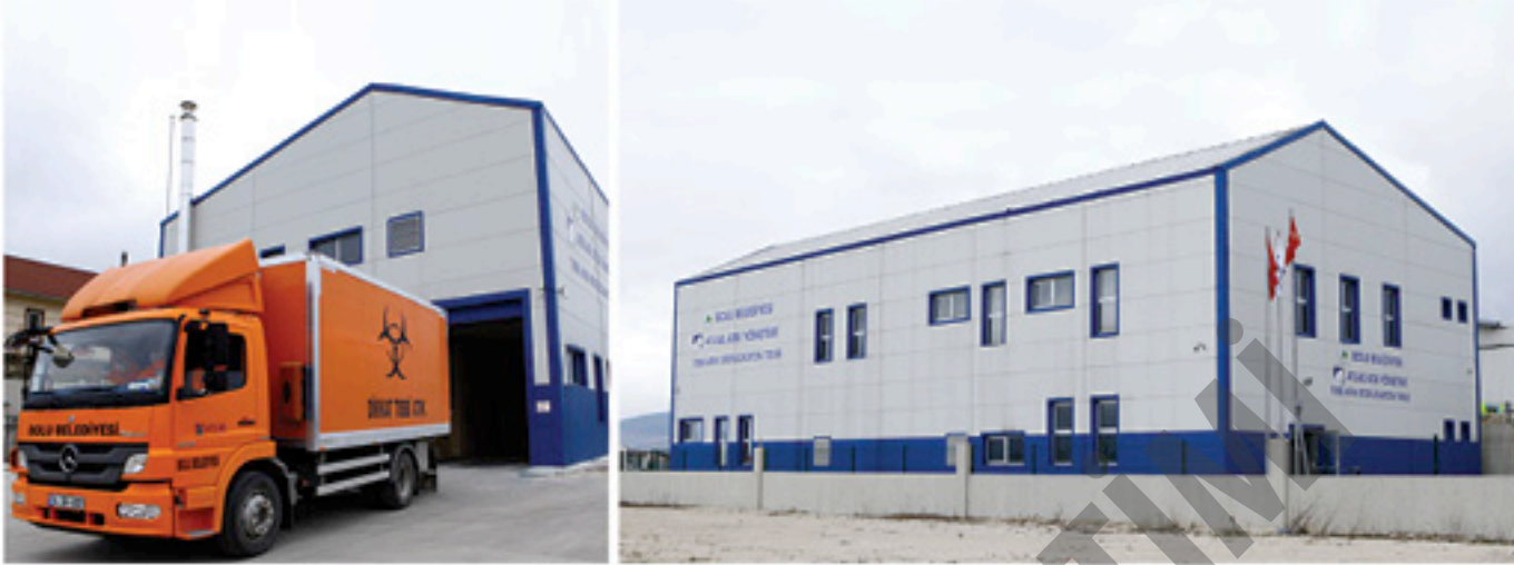
BOLU TIBBİ ATIK TESİSİ / BOLU MEDICAL WASTE FACILITY
